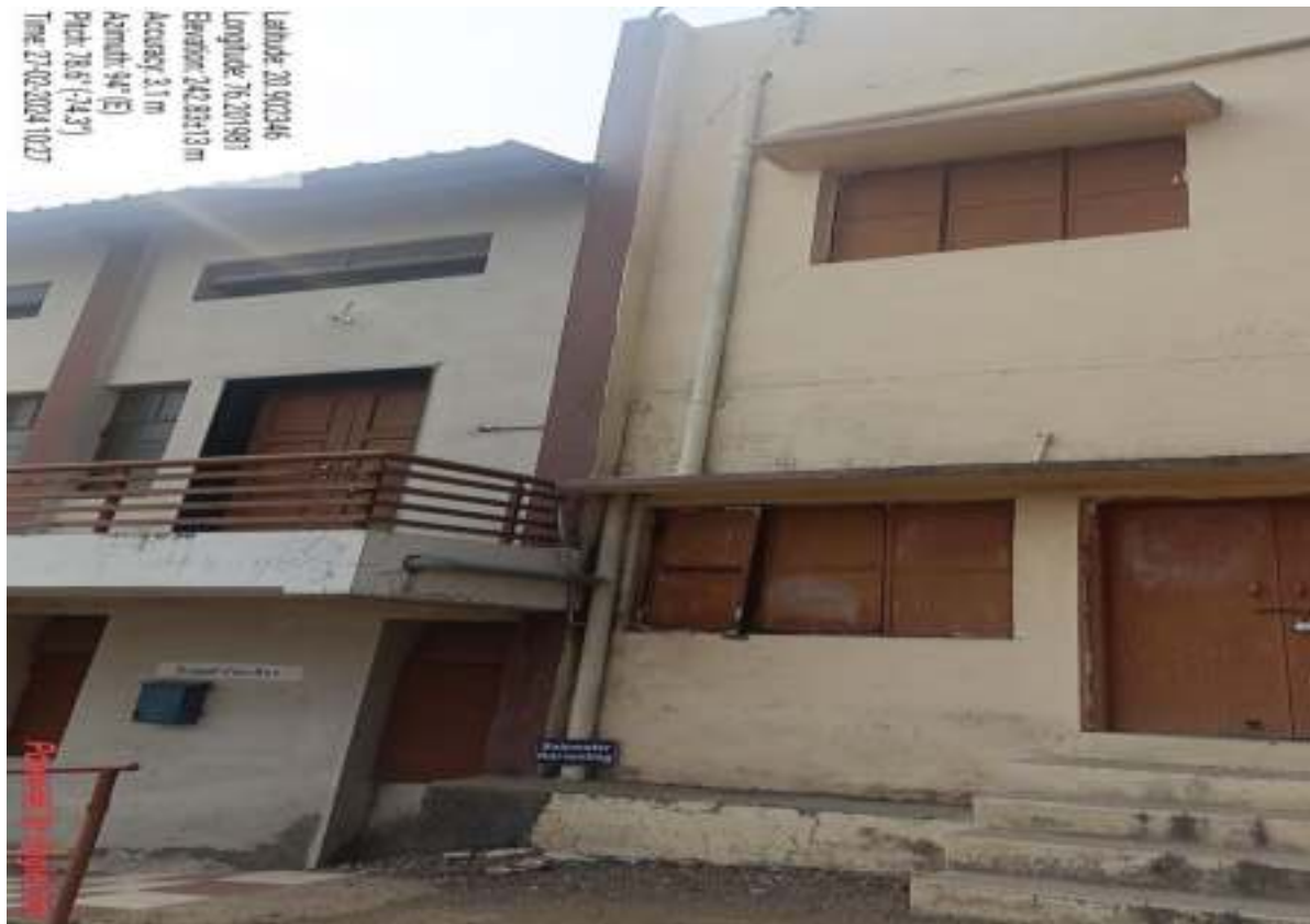
Rain water harvesting
